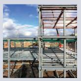
Buildings are designed for 100 years but on average replaced much sooner, and the steel could be re-used, as in this temporary structure.
